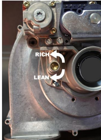
Illustration 2 - Air/Gas Mixture Ratio Screw
